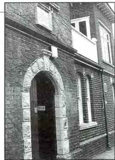
The original main entrance to the hospital now tucked away to the side of the building
